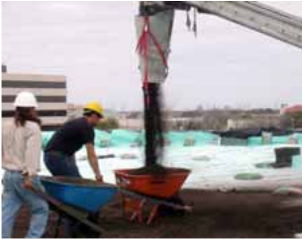
Workers begin to spread the nine inches of soil used on the roof of 251 Medical Center Boulevard.
